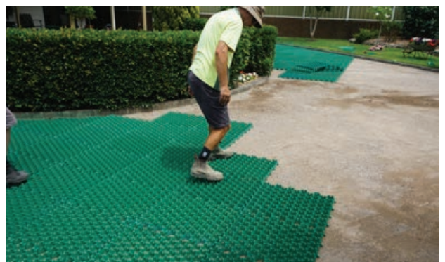
Laying out Econogrid 40 porous pavers
