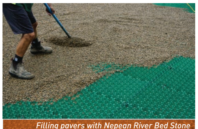
Laying out Econogrid 40 porous pavers
